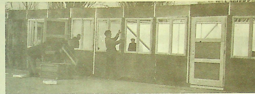
Barracks are built for numerous disaster victims at Zimnicea.
